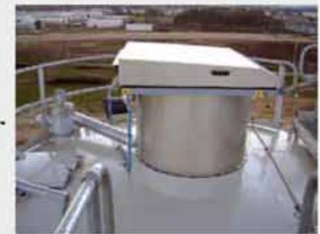
Filtration surface area: 1 ~ 48 m<sup>2</sup> (11 ~ 517 sq ft) Air volume: 60 ~ 4,500 Nm<sup>3</sup>/h (35 ~ 2,650 cfm)
