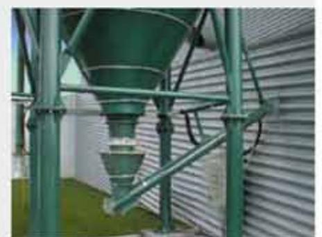
$Q_{\max} = 7 \text{ m}^3/\text{h}$  (4 cfm) For lime dosing plant
